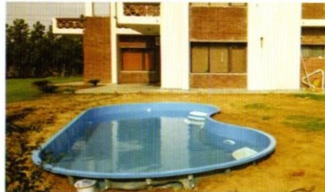
5. Filling water in pool and make deck area.
