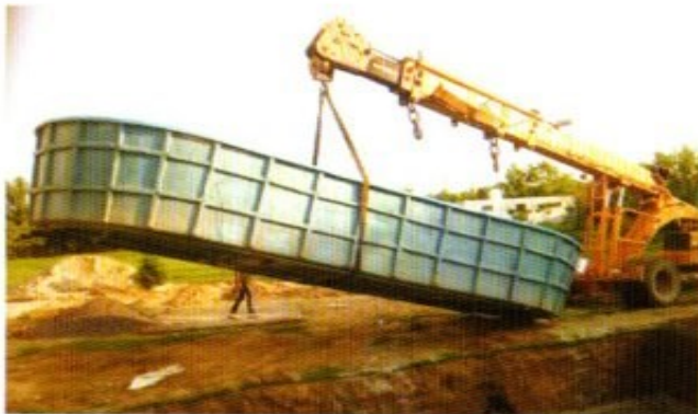
4. Lifting of swimming pool and placing on the prepared floor.
