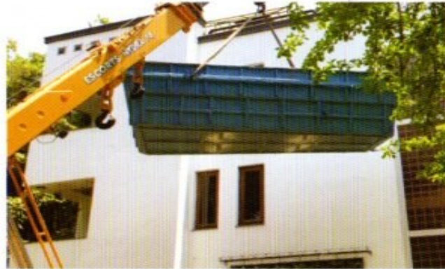
2. Placing the pool with the help of Crane at site.
